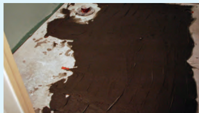
Figure 5 and 6 Installation of a 209 watt floor warming cable in a small basement bathroom. The infrared thermometer shows the formerly frigid basement floor is now a comfortable 25C.
