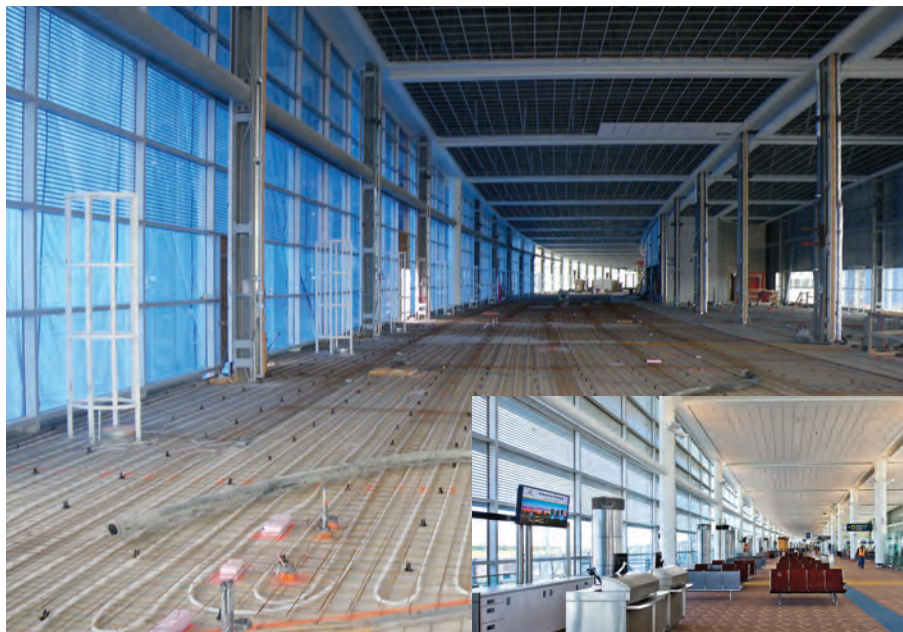
The optimal heated floor zone placement was within a 25-foot deep band from the foot of the curtain wall. During and after construction shown here.
